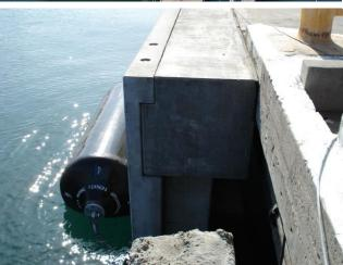
Upgrades to the homeport were completed in 2006. These upgrades included the installation of 5 ft diameter x 12 ft long **Ocean Guard** ™ Netless foam filled fenders. These resilient tough marine fenders are constructed with a heat laminated energy absorbing resilient foam core; a thick tough filament nylon tire cord reinforced non-marking urethane skin; and heavy-duty integral swivel end fittings internally connected with a stud-link chain.
